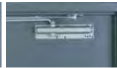
Replacement Plate with NEW door closer installed.
